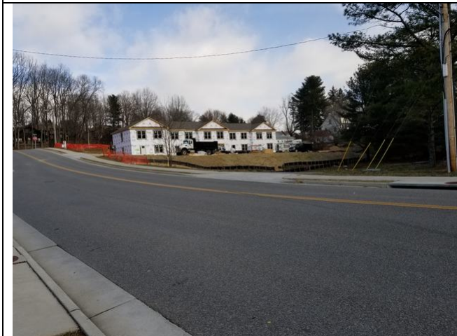
VIEW NORTH OF MARKET RATE TOWNHOMES UNDER CONSTRUCTION ACROSS FROM SUBJECT
