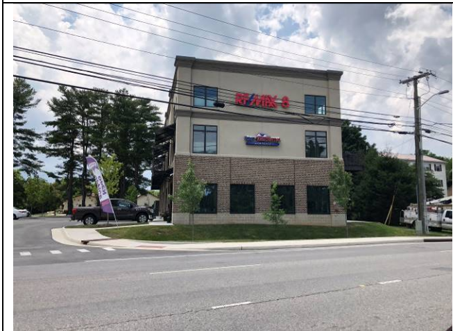
TYPICAL COMMERCIAL USE NEAR SUBJECT
