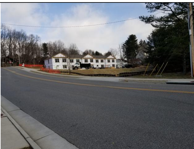
VIEW NORTH OF MARKET RATE TOWNHOMES UNDER CONSTRUCTION ACROSS FROM SUBJECT
