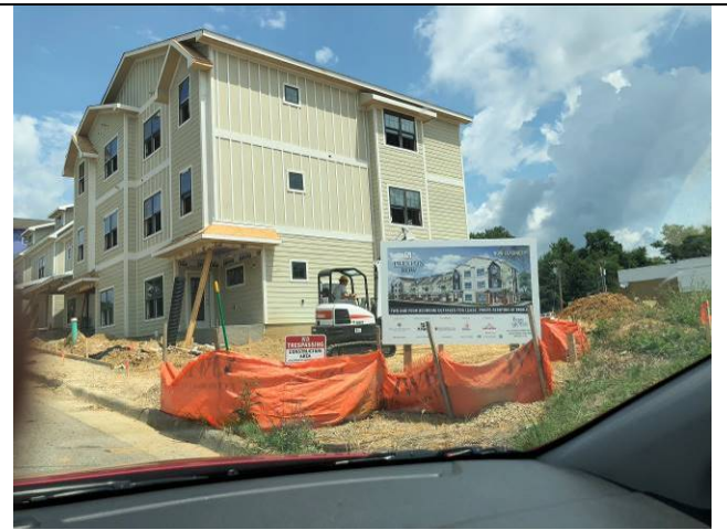
STUDENT HOUSING UNDER CONSTRUCTION NEAR SUBJECT
