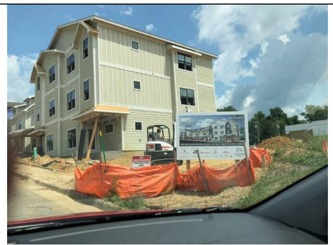
STUDENT HOUSING UNDER CONSTRUCTION NEAR SUBJECT
