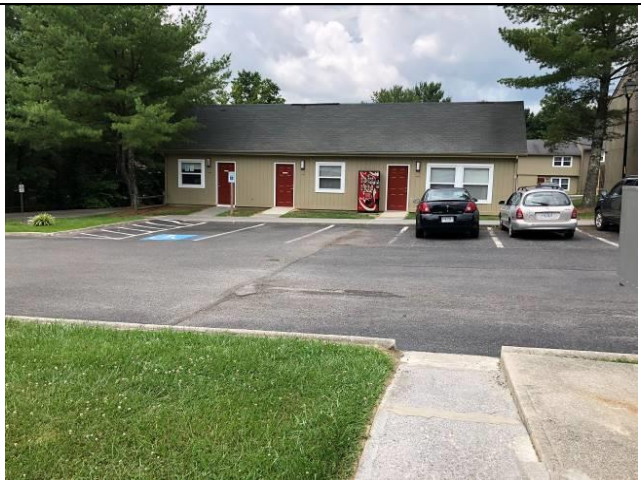
LEASING OFFICE/MAINTENANCE SHED AT SUBJECT
