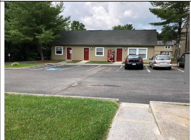
LEASING OFFICE/MAINTENANCE SHED AT SUBJECT
