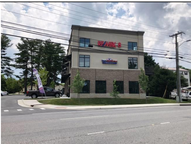
TYPICAL COMMERCIAL USE NEAR SUBJECT
