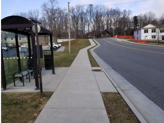
BUS STOP IN FRONT OF SUBJECT
