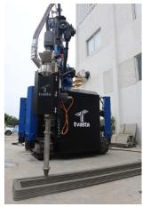
3DCP involves an additive construction process to create concrete structures layer by layer. Unlike traditional construction methods that rely on molds and manual labor, 3DCP automates the process, allowing for faster, more precise construction with less material waste. This technology is primarily used to build walls, structural components, and even entire buildings.
