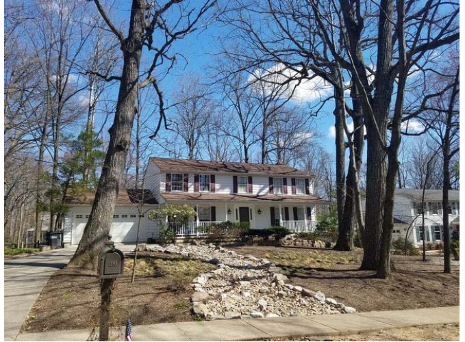
Single-family home east of the Subject site
