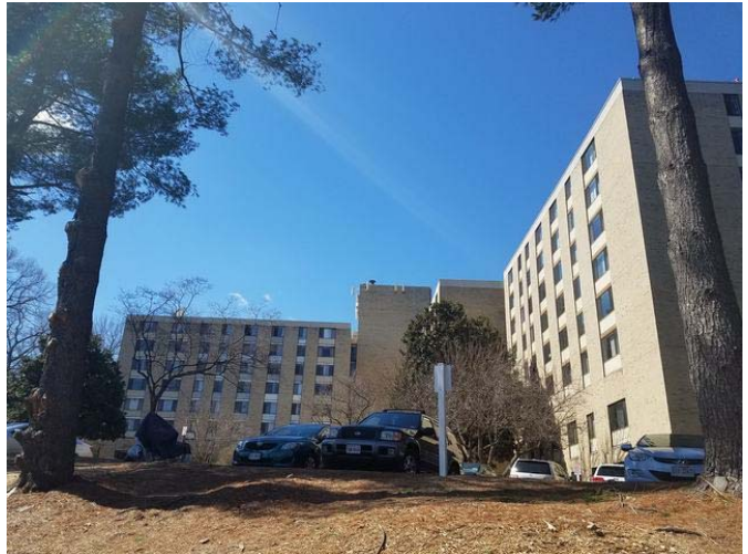
Existing Lake Anne Fellowship House I and II adjacent west of the Subject site (to be demolished)
