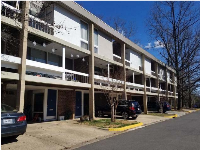
Condominiums west of the Subject site
