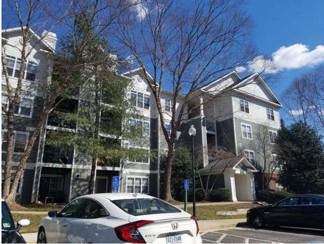
The Apartments at Harbor Park north of the Subject site (excluded – more comparable properties available)
